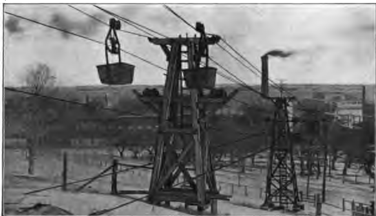
Length of line, 16,500 feet. BLEICHERT TRAMWAY, Hourly capacity, 75 tons. Built by THE TRENTON IRON CO., Trenton, N. J., For the Solvay Process Co., Syracuse, N. Y. View showing wood and iron supports.
