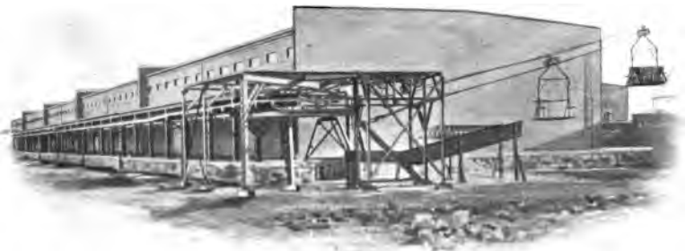
Length of line, 1,150 feet. WIRE ROPE TRAMWAY, Hourly capacity, 7\frac{1}{2} tons. Built by THE TRENTON IRON CO., Trenton, N. J., For the Plymouth Cordage Co., Plymouth, Mass. View of angle station.
