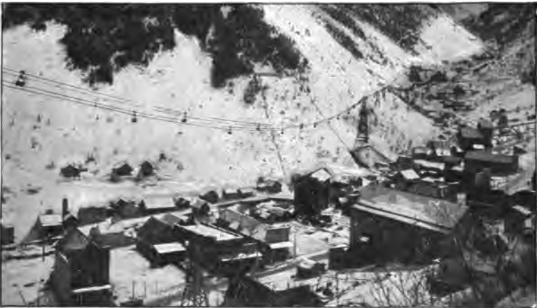
Bleichert Tramway of the Bunker Hill and Sullivan Mining and Concentrating Company. Showing long span across the town of Wardner, Idaho.
