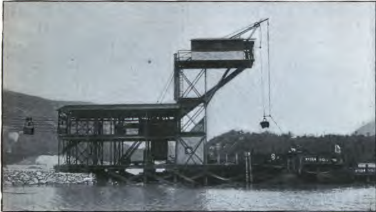
Length of line, 1,640 feet. BLEICHERT TRAMWAY, Hourly capacity, 37\frac{1}{2} tons.
