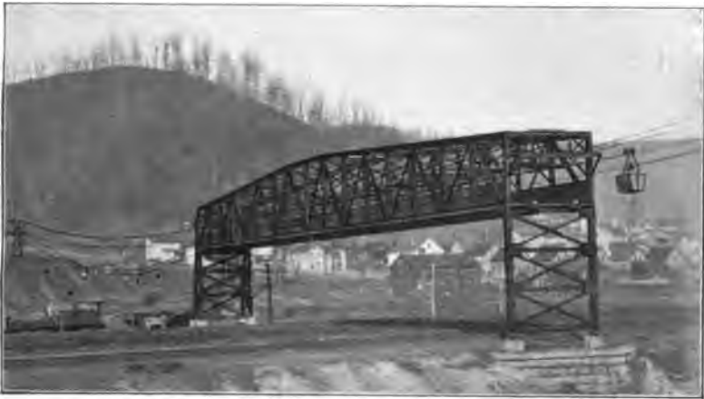
Length of line, 3,260 feet. BLEICHERT TRAMWAY, Hourly capacity, 50 tons. Built by THE TRENTON IRON CO., Trenton, N. J., For The Cambria Steel Co., Johnstown, Pa. View of guard-bridge across the Pennsylvania R. R.
