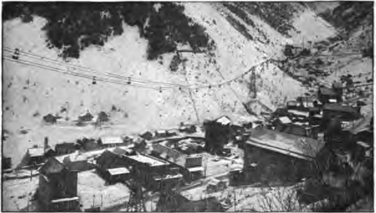
Bleichert Tramway of the Bunker Hill and Sullivan Mining and Concentrating Company. Showing long span across the town of Wardner, Idaho.
