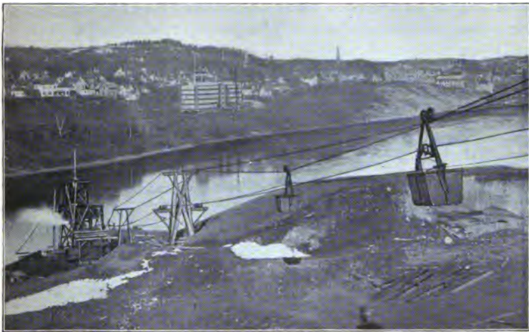
Length of line, 1,050 feet. BLEICHERT TRAMWAY, Hourly capacity, 30 tons.
