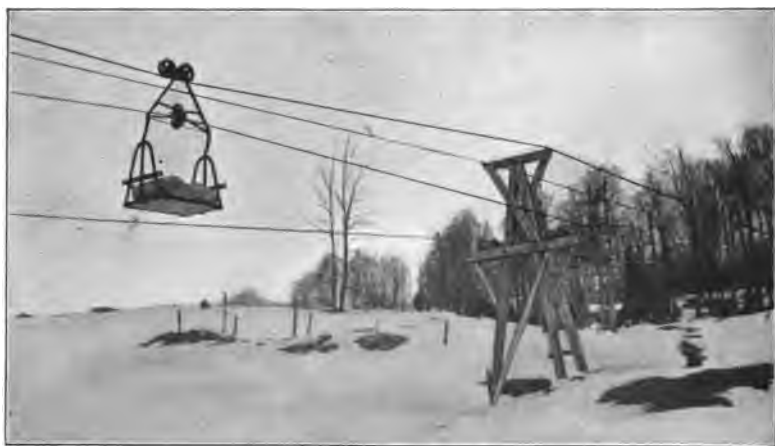
Length of line, 2,400 feet. BLEICHERT TRAMWAY, Hourly capacity, 2½ tons. Built by THE TRENTON IRON CO., Trenton, N. J., For The New England Talc Co., Stockbridge, Vt., showing platform car.
