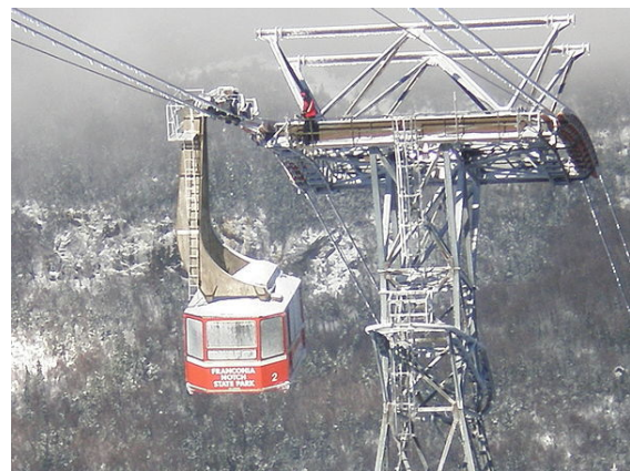
Routine maintenance at the upper tower
