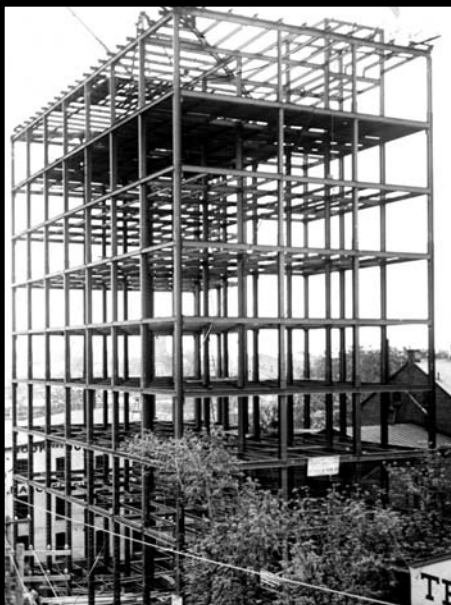
Figure 18: Broad Street Bank Building, 1899. The New Jersey Steel & Iron Company erected the steel frames of many prominent buildings, including Trenton's first skyscraper. Trenton Public Library.
